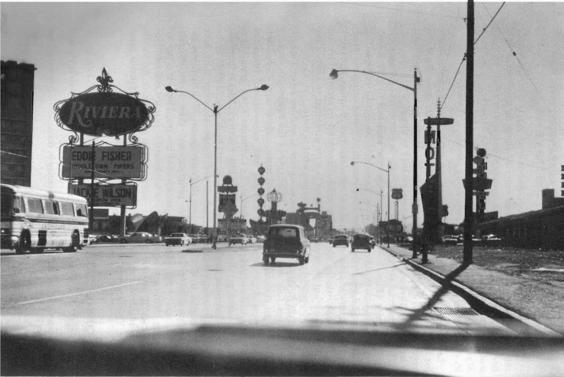
The Las Vegas Strip, looking southwest
